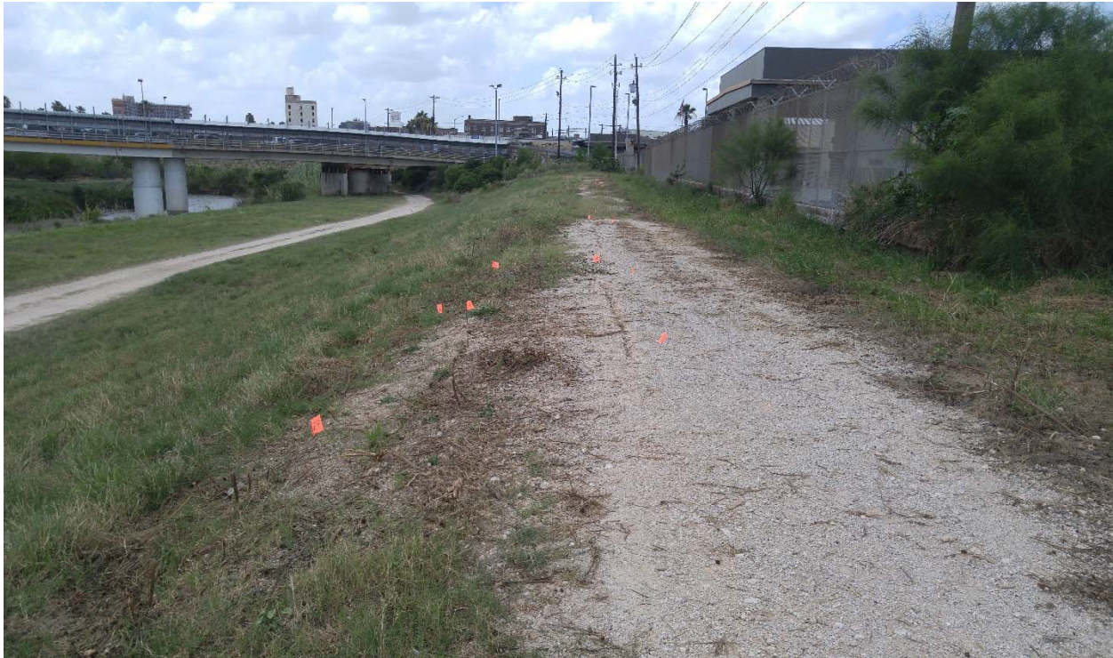
Photo 3 - Looking North - Surface Tension Crack of Pin Flags 11B through 20B.
