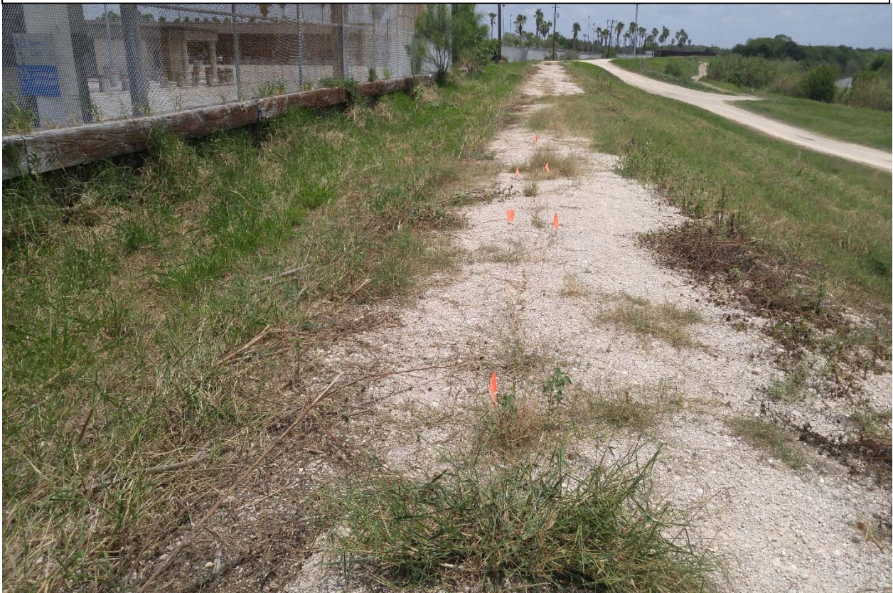
Photo 2 - Looking South - Surface Tension Crack of Pin Flags 5B through 10B
